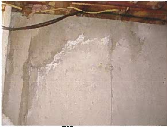
Efflorescence
